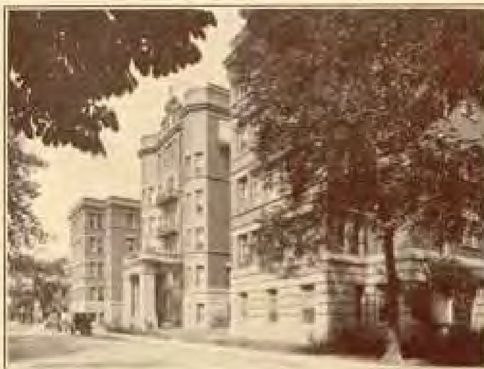
MINISTRE SAINT-MARC'S—A VIEW OF BUILDING FROM THE STREET AND GARDEN.
