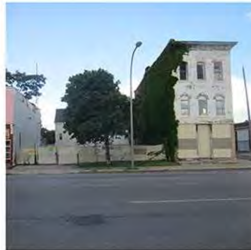
1227 (Parking Lot) and 1225 Niagara Street
